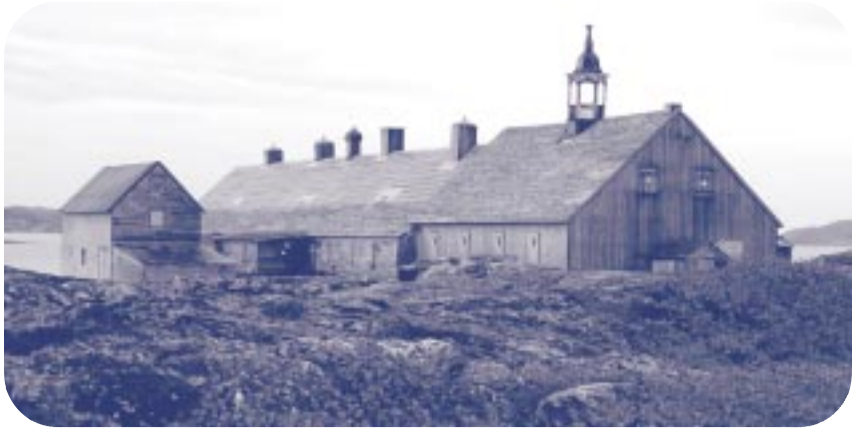
Photo: Hebron Restoration Site.
