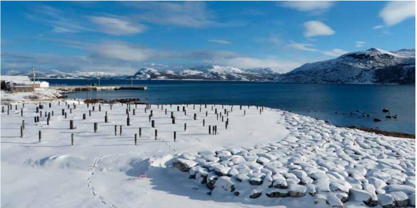
**Phase one of construction includes a breakwater, building area site work, and drilling and installation of piles.**
